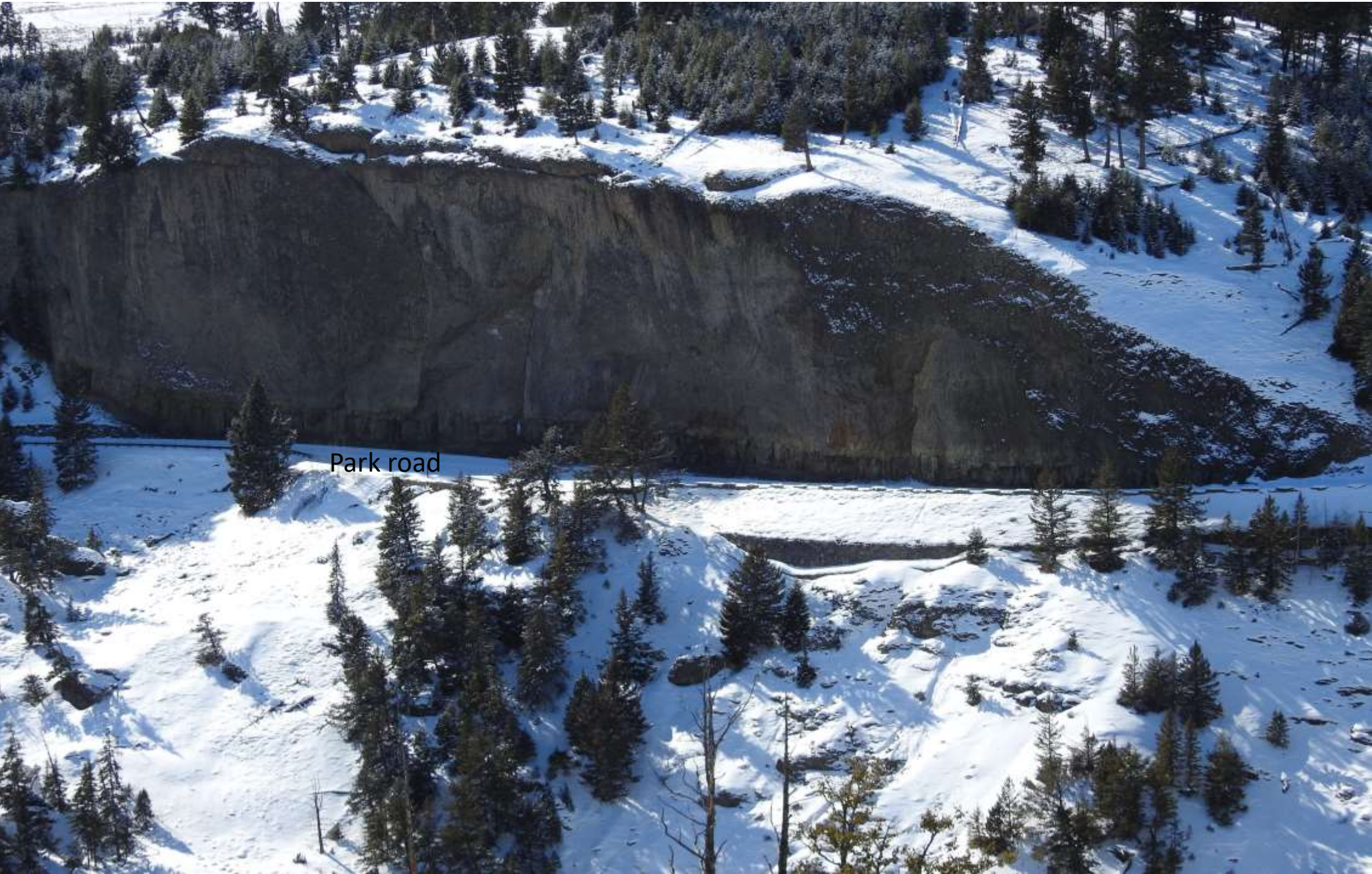
Cliff above the park road near Tower Fall.
