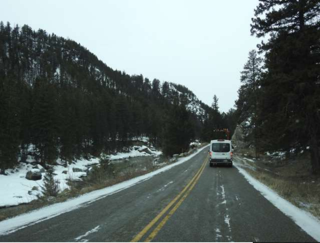
Lamar Canyon with the Lamar River (left) and the one lane portion of the road (right). The area to the right was blasted in summer 2023 to make the road wider and further away from the cliff above the river.
